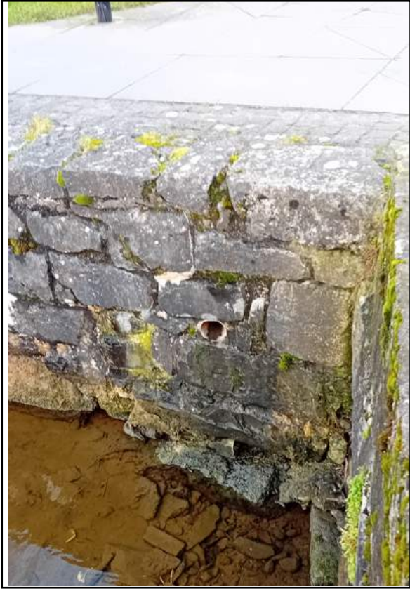
Gully trap outfall at Waterside
